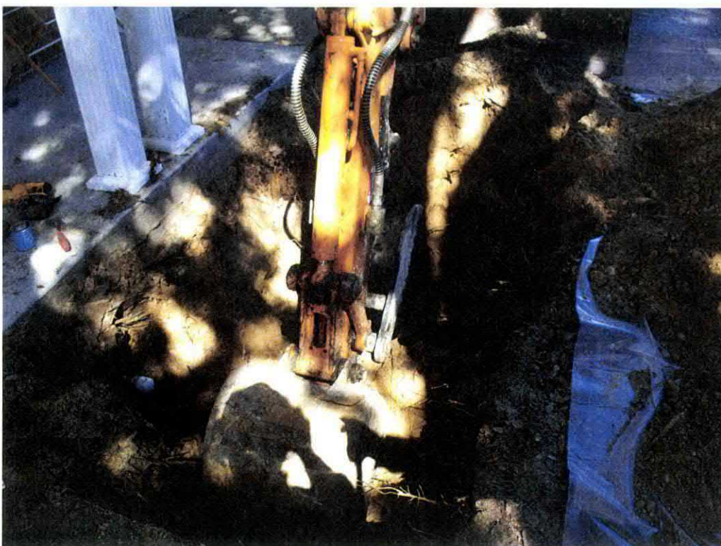
Picture 2: UST 368Aspen removal in progress.
